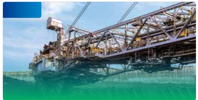
Mines: Main ventilation fans, pressurised fans, extractor fans, air compressors, pumps, belt conveyors, mills, etc.
