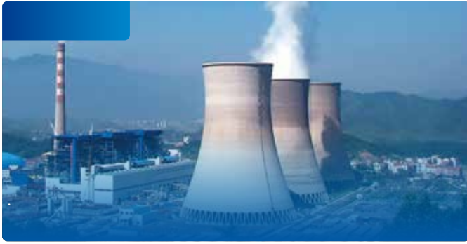
Thermal power generation: induced draft fan, supply fan, dust-absorbing fan, booster fan, compressor, condensate pump, feed water pump, make-up water pump, grey slurry pump, and so on.
